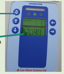
Mute buttons can be in different places (within the  $O_2$  monitor panel itself or in a more comprehensive wall display panel). Know the difference between an oxygen sensor alarm and a chiller fault alarm.
